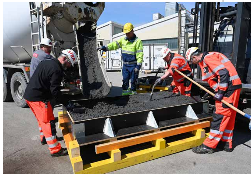
Climate-friendly concrete was tested in summer and winter trials. © Doka
