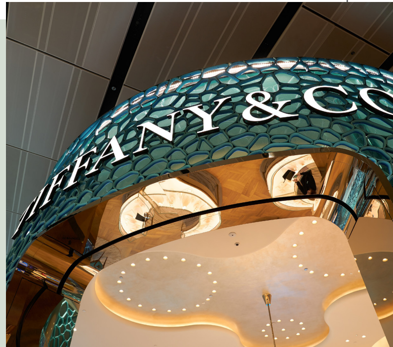
Manufacturer Aectual supplied the stunning 3D-printed facade made from recycled marine debris for the Tiffany’s boutique at Singapore’s Changi Airport. © Shutterstock: Sorbis
