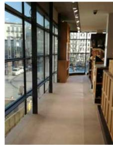
For Manufactum in Hannover the gallery was closed off with special steel sections to enlarge t sales area. The ceiling ends flush with the windows, extending them down to the floor.
